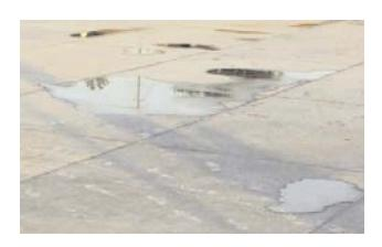
Expecting or requiring no birdbaths on level or sloped slabs is not compatible with ACI 117 tolerances. Specifying a relatively large permissible gap under a straightedge (low  $F_F$ ) results in numerous deep birdbaths. Specifying a small gap under a straightedge (high  $F_F$ ) results in a few shallow birdbaths.
