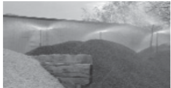
Sprinkling Aggregate in a Stockpile
